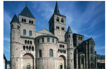
Liebfrauenkirche (Cultural Heritage) Trier, Germany
