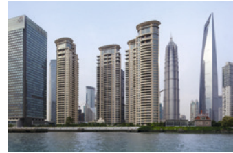
Tomson Riviera Apartment Towers Shanghai, China
