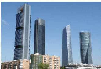
4 Towers Business Area Madrid, Spain
